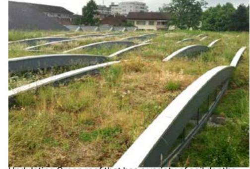
Undulating Green roof that has a variety of soil depths.
