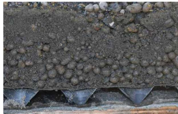
Green roof substrate cross section
